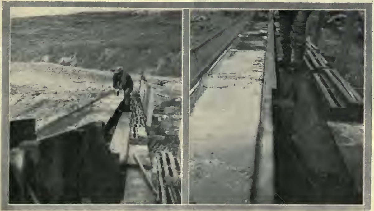
PREPARING TO CLEAN-UP.
